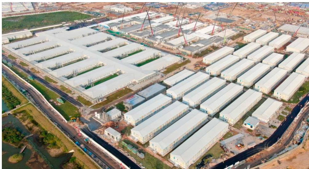
Construction of Central Government-Aided anti-pandemic facilities completed in Hong Kong on May 6, 2022 in 51 days, making it a milestone for constructing a mega project in such a short period of time.
