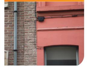
This cable has a capacity from 24 to 96 fibres. Access to the fibres by window cut is quick and easy thanks to a flexible UV resistant sheathing material. Each units can be pulled back on more than 1m to easily connect the facade distribution box.
