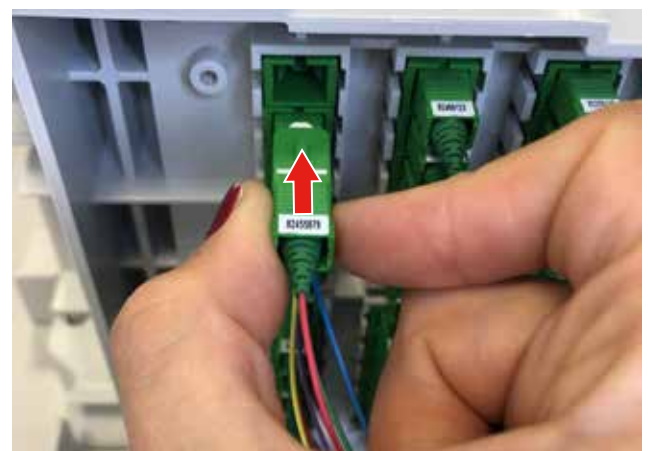
5 Reconnecter le pigtail et le cordon Reconnect the pigtail and the patchcord
